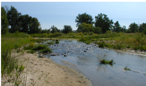
Photo showing restored stream with riffle drop just after construction.
