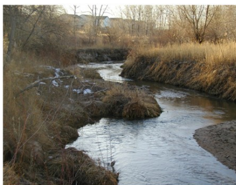
Degradation had lowered the project reach approximately 5-feet below the adjacent top of banks, exposing two sanitary sewer crossings.
