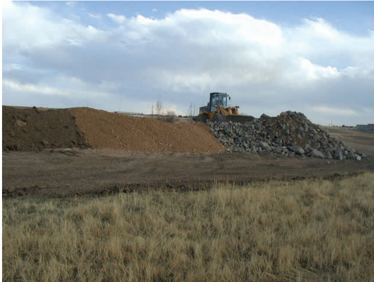
Stockpiles of the separate void-fill materials.
