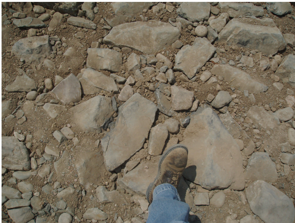
Void-filled riprap after placement and compaction.
