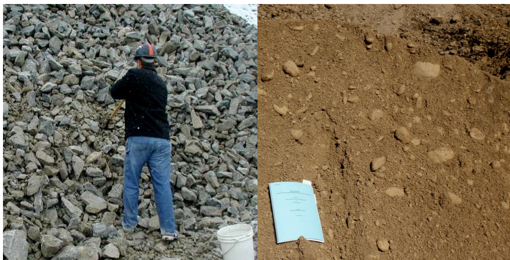
Two key ingredients to fill in the gaps between riprap pieces are 7-inch minus crushed surge (left) and 4-inch minus pit run surge (right)
