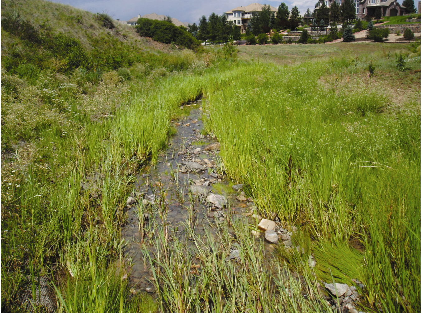
The Upper Marcy Gulch void-filled riprap lining project has created a stable, well vegetated stream to reclaim the former eroding, incised gulch.
