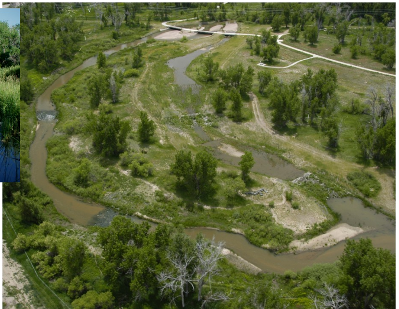
Aerial perspective photo of Cherry Creek Open Space Restoration Project soon after construction showing riffle drops and secondary channel under high Spring flows.
