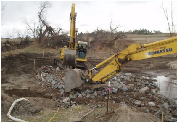
Void-filled riprap often needs to be re-mixed in place to maintain a uniform distribution of particle sizes.
