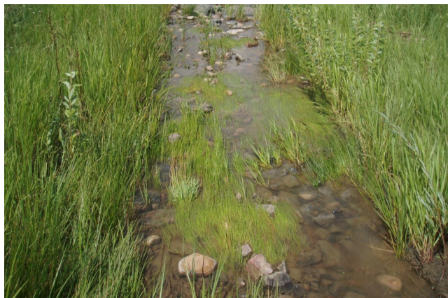
This photo attests to the ability of void-filled riprap lining to support wetland and riparian vegetation and keep flows on top of the rock.
