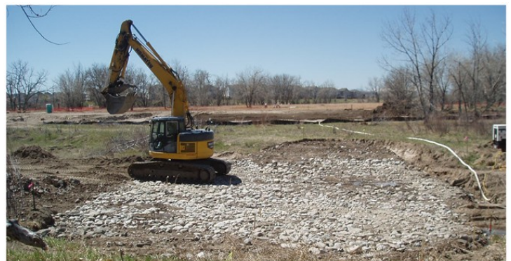
Photo showing smooth layout of void-filled riprap after compaction by excavator.
