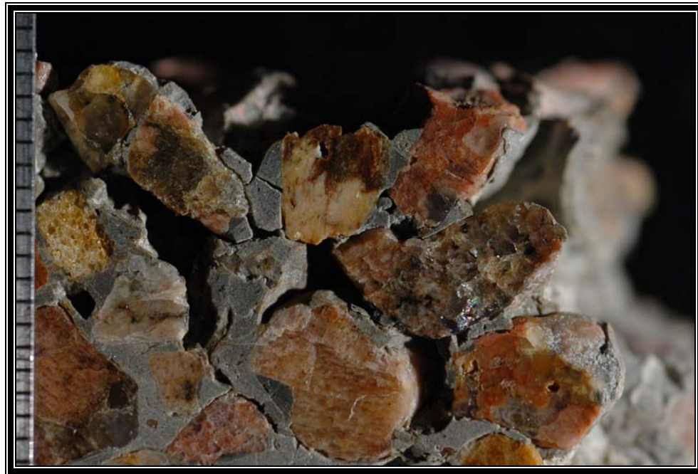
Figure B3. (a) Photograph of polished surface showing overview of cracking near the top of the slab; scale in millimeters.
