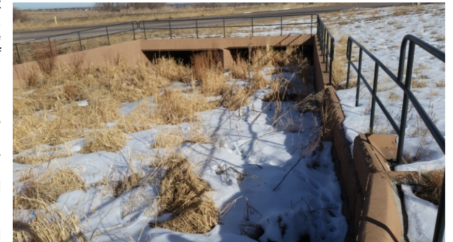
Photo 3: MDP Reach WC-3 – Existing Crossing Underneath Quincy Avenue
