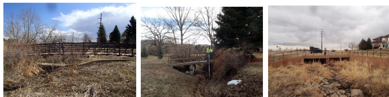
Channel Manning's "n" = 0.05 Channel Manning's "n" = 0.05 Channel Manning's "n" = 0.07 Overbank Manning's "n" = 0.05-0.1 Overbank Manning's "n" = 0.04-0.045 Overbank Manning's "n" = 0.05
