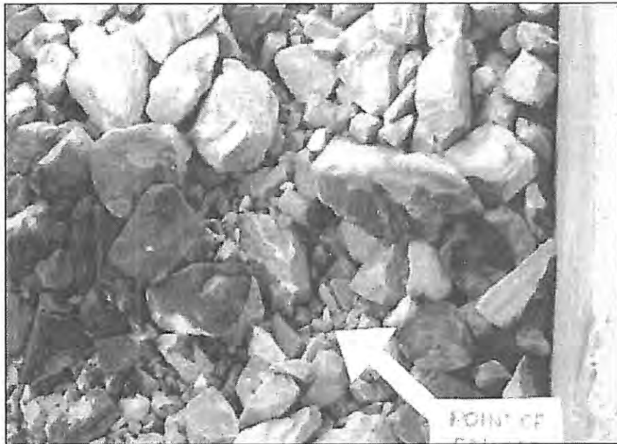
Figure 5.9. Riprap failure in 1997 tests ( d_{50} = 0.89 ft (271 mm)).
