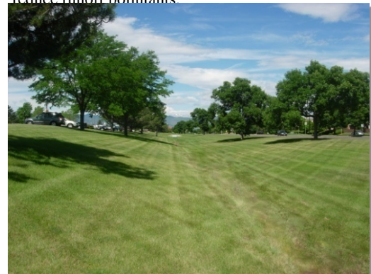
Photograph 1-3. Grass Swale. This densely vegetated grass swale is designed with channel geometry that forces the flow to be slow and shallow, facilitating sedimentation while limiting
