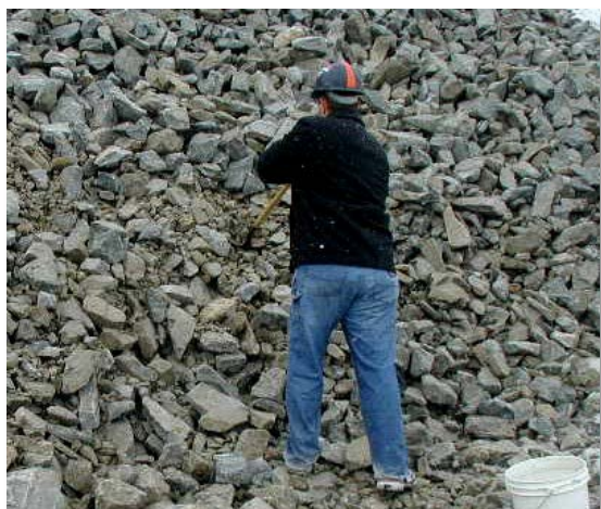
Photograph 8-19. Seven-inch minus crushed surge is a key ingredient to fill gaps between riprap.
