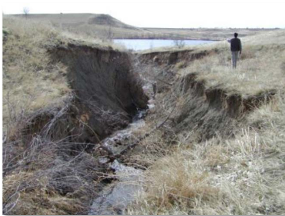
Photograph 8-7. Degraded channel (before restoration).
