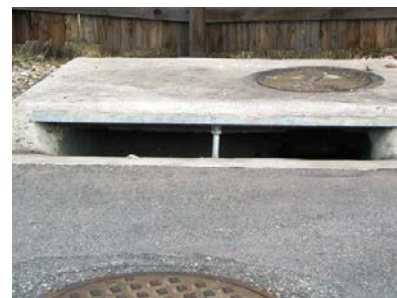
(c) CDOT Type R curb-opening inlet
