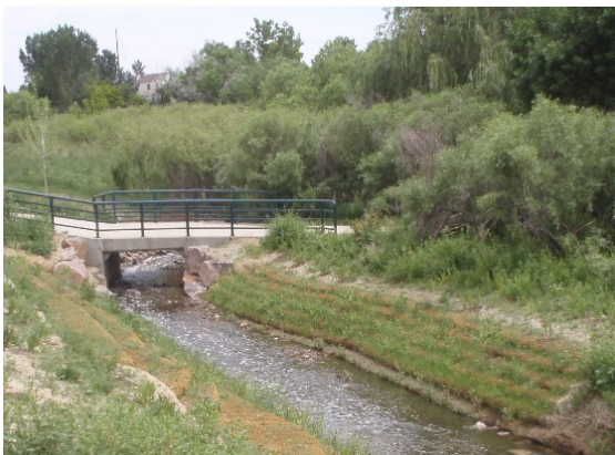
Photograph 8-15. Soil lifts used to stabilize banks of low-flow channel. Photo taken immediately after construction.
