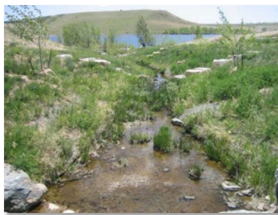
Photograph 8-8. Same channel as photo 8-7 after restoration.
