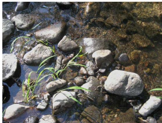
Photograph 8-18. Void-filled riprap is designed to emulate natural riffles, consisting of a mix of rock, gravels and sands that is densely-packed and able to support riparian vegetation.
