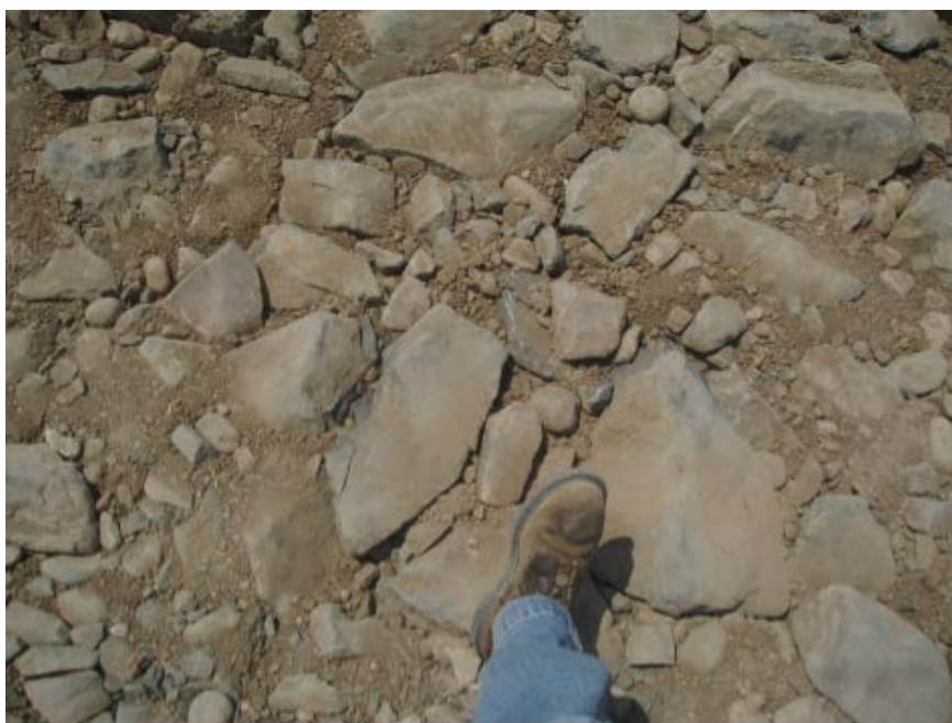
Photograph 8-21. Void-filled riprap after placement and compaction.
