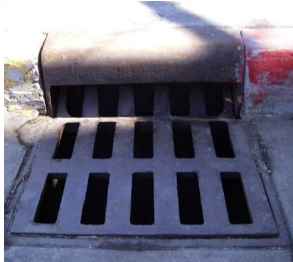
Raccoons inhabiting storm drain system (a) and retrofitted storm drain inlet (b). (Photos courtesy of City of Boulder, Colorado)
