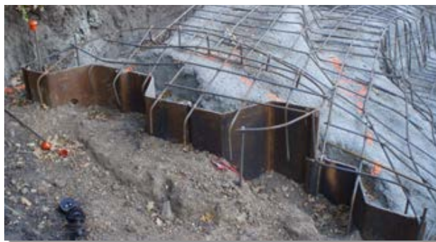
Photograph 9-4. View of the sheet pile cutoff wall and steel reinforcement for a sculpted concrete drop structure prior to the concrete placement. Note the steel reinforcement has been spot welded to the sheet pile.
