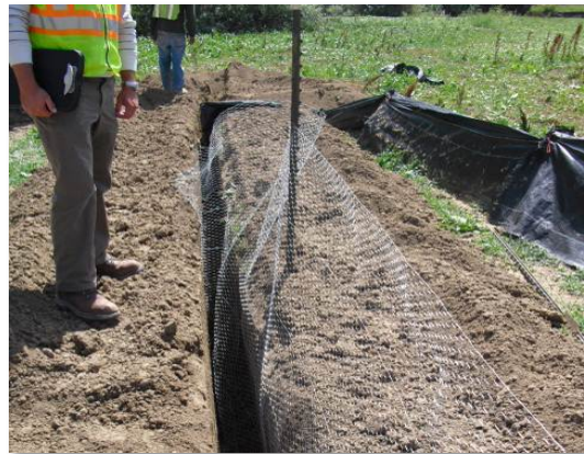
Photograph 13-7. Prairie dogs will attempt to dig under the fence. Bury the wire mesh portion vertically (shown) or in the form of an “L” to deter prairie dogs from burrowing under the fence.
