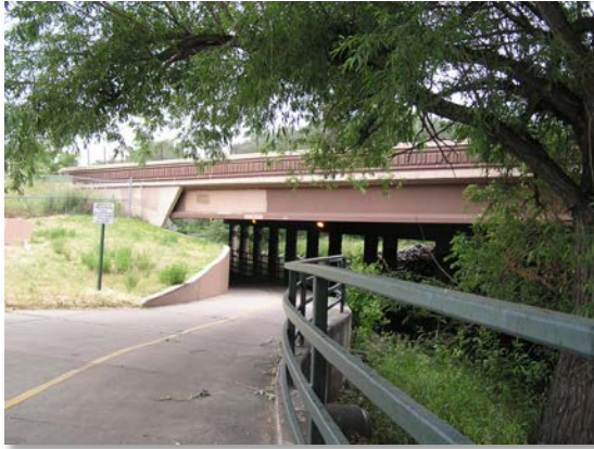
Photograph 10-7. Horizontal members are placed on the users' side of the posts. This is an important consideration for both shared-use paths and equestrian trails in that it reduces the chance of snagging clothing, a bike pedal or a stirrup.
