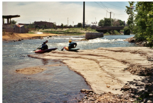
Photograph 10-41. This sculpted concrete jetty forms a small eddy downstream to enhance access to the river. The sculpted concrete surfacing also provides for direct access into the water’s edge. Photo courtesy of McLaughlin Whitewater Design Group.
