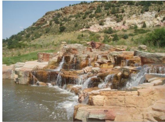
Photograph 9-24. Stained concrete in foreground with natural rock in the background.
