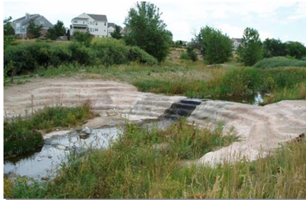
Photograph 9-9. A sculpted concrete drop structure along Marcy Gulch in Highlands Ranch, CO represents a basic structure design.
