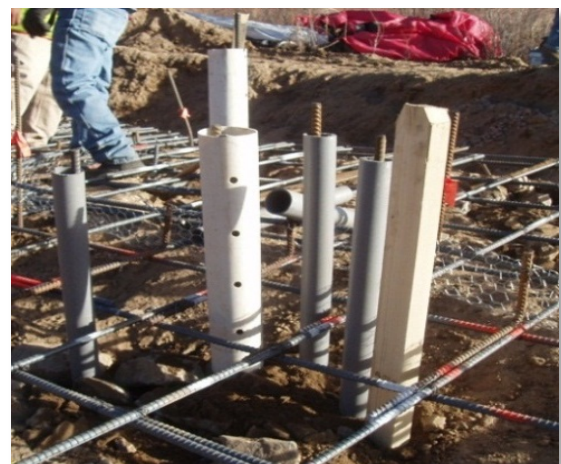
Photograph 9-17. Small vegetation pockets can be formed using PVC, lumber, or other items. Removed these items shortly before or after the concrete cures. If done after the concrete cures, coat the items with a lubricant to facilitate removal.
