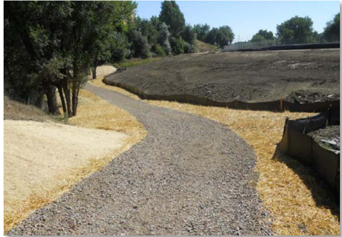
Photograph 10-25. This stabilized rock trail was constructed for maintenance.
