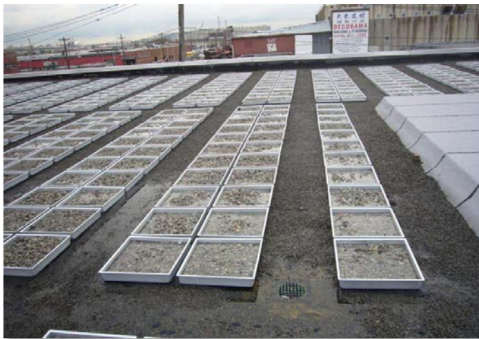
Photograph 12-4. This blue roof system utilizes trays. The design appears as an intentional feature to the lay person. Additionally, the design is such that it cannot be easily manipulated. Photo courtesy of Geosyntec.
