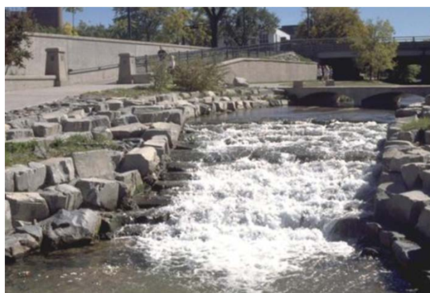
Photograph 9-5. Example of stepped downstream face for a grouted boulder drop structure. Note dissipation of energy at each step for low flows.
