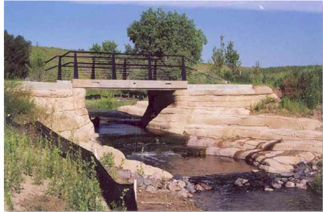
Photograph 11-5. Shared-use path over Grange Hall Creek.
