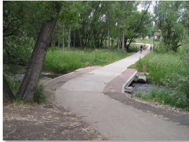
Photograph 10-21. A Bear Creek cast-in-place concrete culvert crossing with rumble strips and a crossing with rails in the distance.
