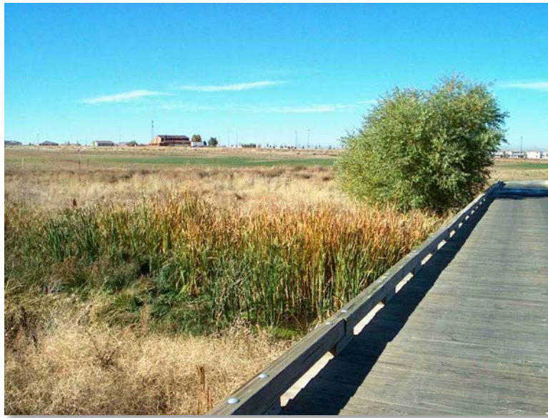
Photograph 10-6. Curb rails are typically no higher than 12 inches and can be constructed from a variety of materials.
