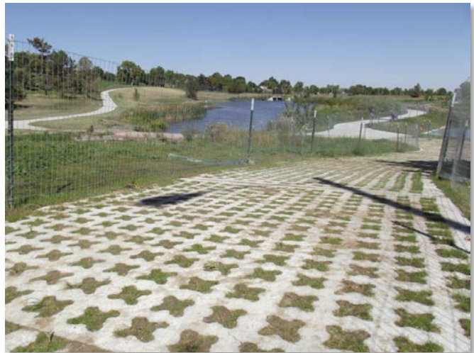
Photograph 10-26. Reinforced grass pavement shortly after construction.
