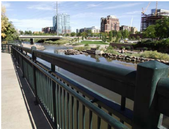
Photograph 10-8. At Confluence Park a rubber rail was included as part of the rail design. This, in addition to the 14-foot path width, improves safety in this high-use area.
