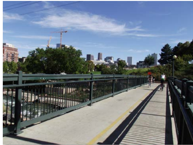
Photograph 10-22. A pedestrian bridge crossing with rails at Confluence Park.
