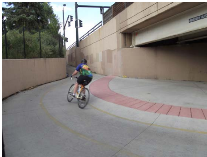
Photograph 10-13. Understanding the popularity of the Cherry Creek path, designers worked to make the underpass at University safe for bicyclists and pedestrians while working within the limitations of the existing site. Land was purchased to create a suitable turning radius at this 90 degree bend. This provides bicyclists with additional time to react to the unexpected.
