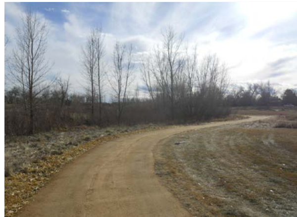
Photograph 10-28. StaLok® paving material, a proprietary surface consisting of resin bound gravel, has replaced failed portions of the crusher fines Goldsmith Gulch path.
