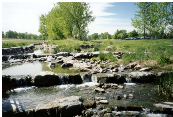
Photograph 9-2. Grouted stepped boulder drop structures such as this one in Denver’s Bible Park can be safe, aesthetically pleasing, and provide improved aquatic habitat besides performing their primary hydraulic function of energy dissipation.
