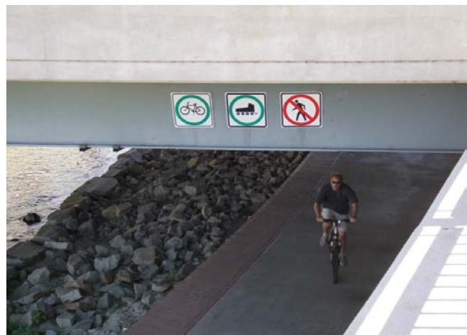
Photograph 10-3. Signing and striping help segregate bicyclists and pedestrians at Confluence Park where the two treads are separated by the creek.
