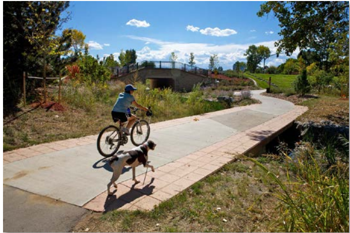
Photograph 10-19. A cast-in-place concrete culvert crossing with rumble strips. Photo Courtesy Architerra Group.
