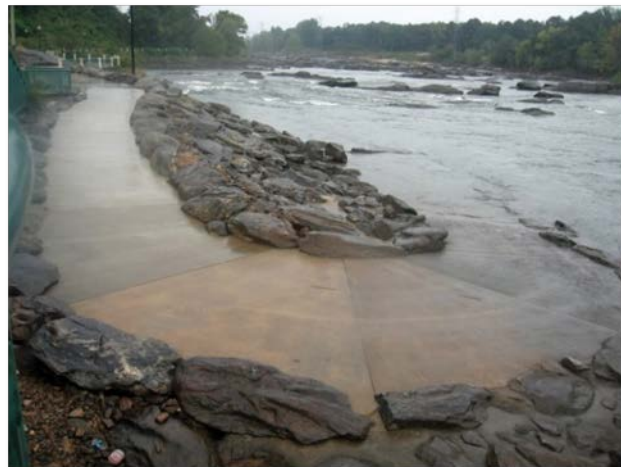
Photograph 10-42. This access ramp was designed with universal access in mind. Photo courtesy John Anderson.
