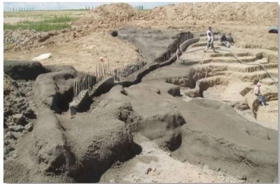
Photograph 9-25. An example of a “skim coat” applied to the prepared subgrade.
