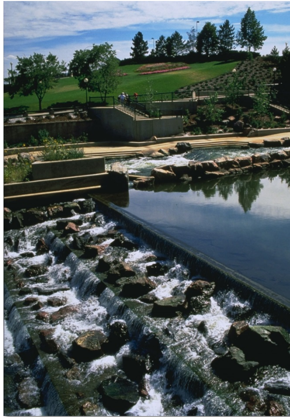
Photograph 10-36. The stepped dam at Confluence Park was physically modeled at multiple flows up to the 100-year event. It was shown to not produce overly-retentive hydraulics throughout this wide range of flows. Photo courtesy of McLaughlin Whitewater Design Group.
