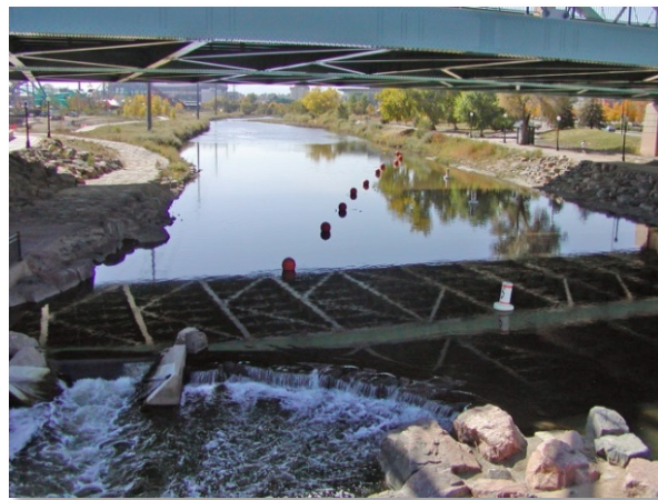
Photograph 10-40. Buoys upstream of Confluence Park Dam guide recreationalists away from the downstream dam and intake. Photo courtesy of McLaughlin Whitewater Design Group.
