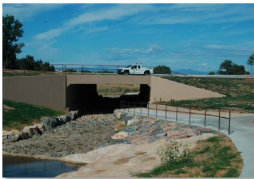
Photograph 10-15. This single-cell three sided box culvert offers safe passage, providing the user with a view of potentially rising water and the path beyond the structure.
