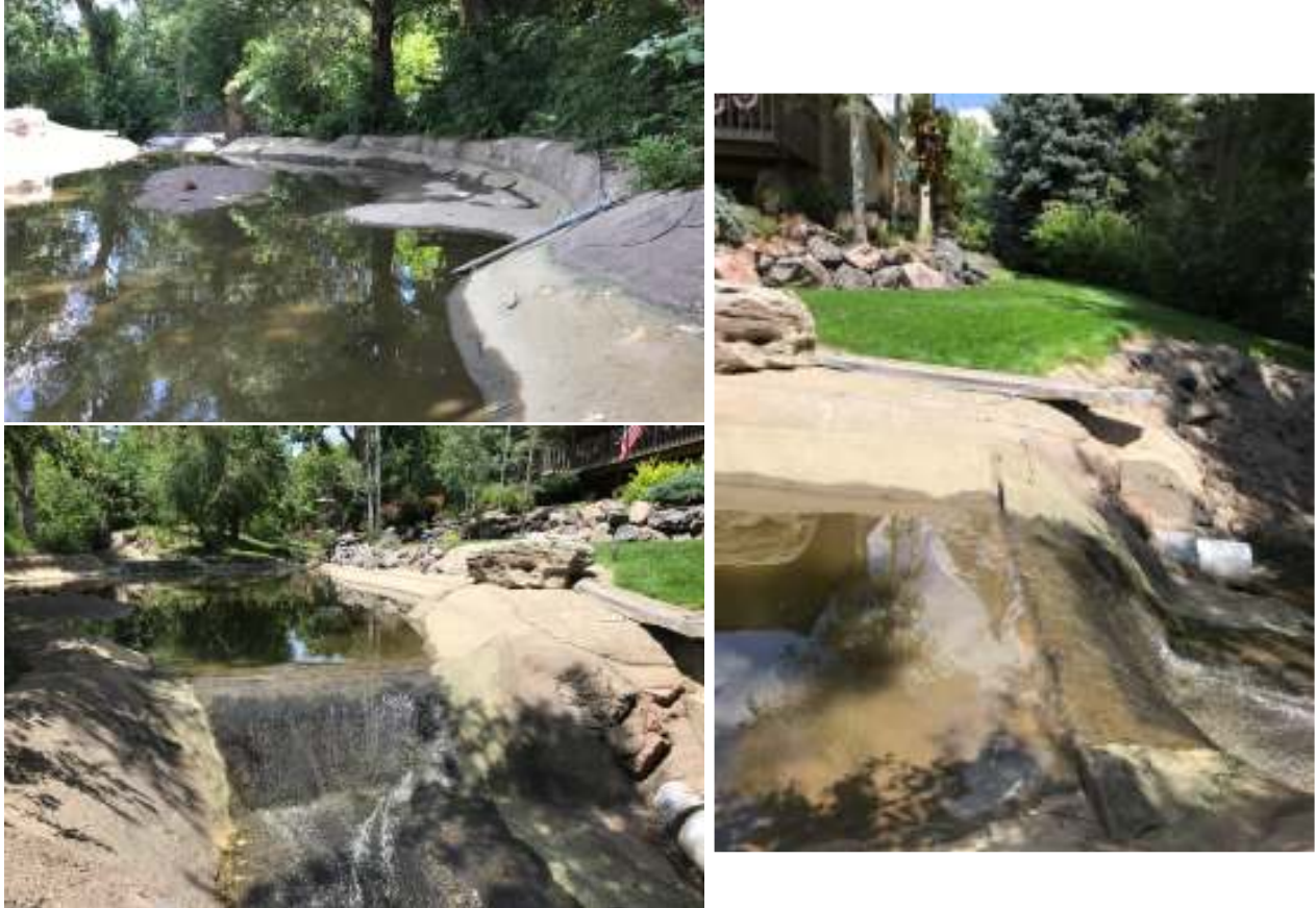
Figure 4. ALERT 1023 Lena @ Nolte Pond, looking downstream, looking upstream at the control and looking at the control and short metal wall (flashboard) lying near the lawn that can be removed.
