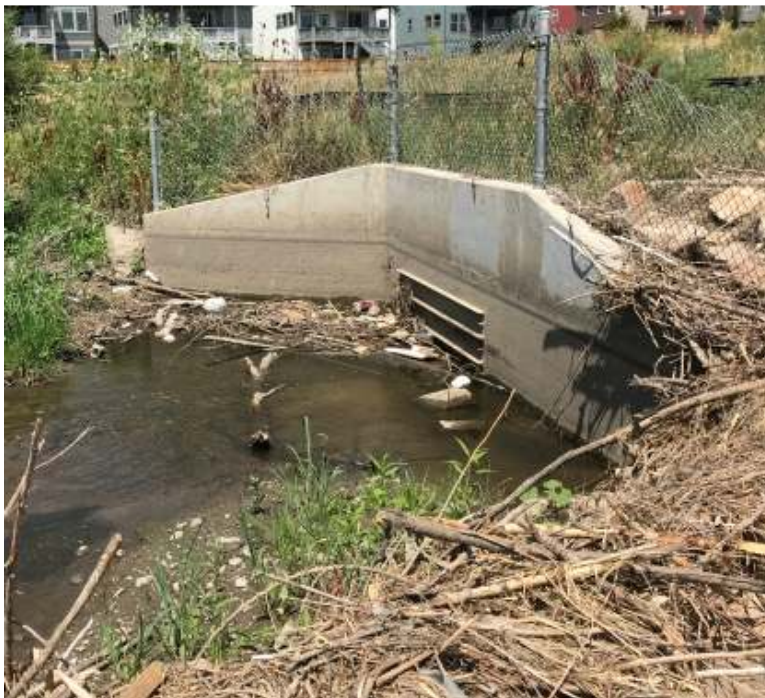
Figure 4. Flood Diversion Structure (circled in yellow on first photo above) 0.5 mi upstream of ALERT Station 1310 (station location in red in first photo above). Culvert/debris dam structure (circled in orange on second photo above) is designed only allow low flows to pass and to divert peak flows through energy dissipation channel on west to detention basin below. Low flows are conveyed to the eastern channel through covered ~2-3 ft diameter culvert.
