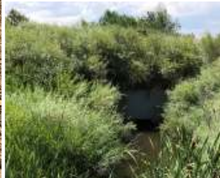
Figure 4. Flood Diversion Structure (circled in yellow on first photo above) 0.5 mi upstream of ALERT Station 1310 (station location in red in first photo above). Culvert/debris dam structure (circled in orange on second photo above) is designed only allow low flows to pass and to divert peak flows through energy dissipation channel on west to detention basin below. Low flows are conveyed to the eastern channel through covered ~2-3 ft diameter culvert.
