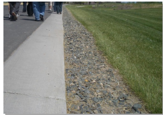
Photograph 1-2. Grass Buffer. This roadway provides sheet flow to a grass buffer. The grass buffer provides filtration, infiltration, and settling to reduce runoff pollutants.
