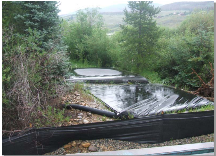
Photograph DW-2. Dewatering bags used for a relatively large dewatering operation.
