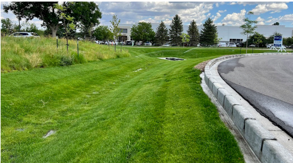
Photograph RPA-2. RPAs including grass buffers and swales treat runoff by filtering and infiltration. For treatment to be effective, grass buffers must receive runoff as sheet flow. Photo: WWE.
