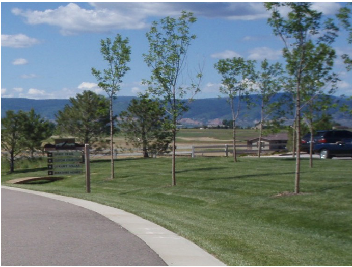
Photograph 4-6. Curbless pavement promotes sheet flow in adjacent grass buffers and swales for filtering and infiltration.
