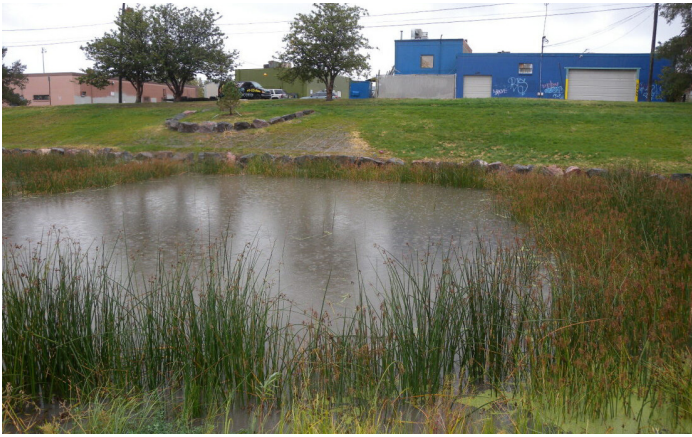
Photograph RP/CWP-4. Landscape elements such as vegetation and stone highlight the irregularly shaped pond edge, making it appear more natural. Photograph courtesy of Design Concepts.
