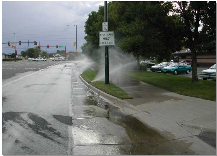
Photograph LM-1. Over-irrigation and overspray can wash fertilizers and lawn chemicals into the storm drain system. These flows can combine with storm runoff and cause nuisance flow conditions in stormwater BMPs. Photo courtesy of the City of Westminster.
