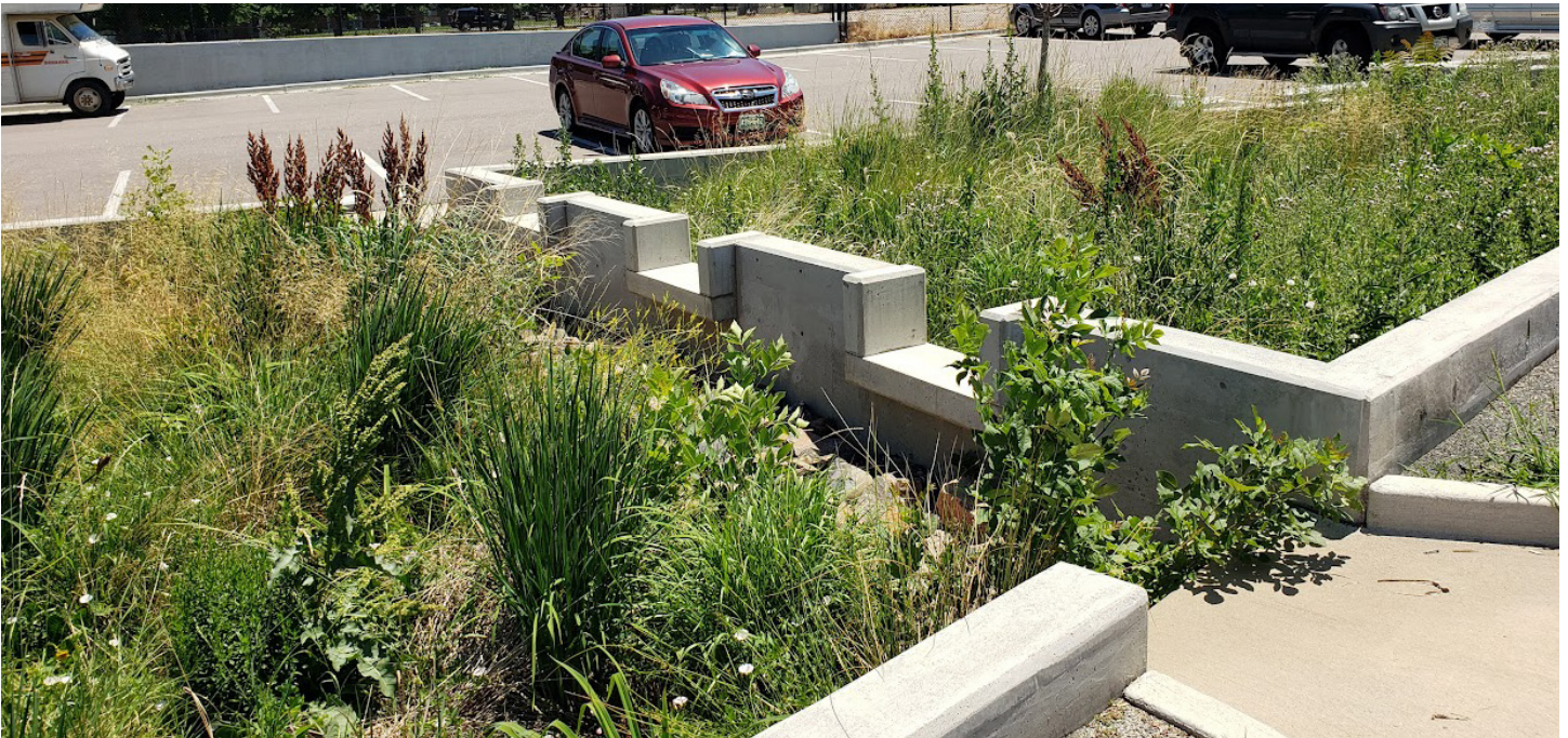
Photograph BR-3. Terraced bioretention SCM in recreation center parking lot. Photo: MHFD
