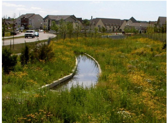
Photograph 4-10. This level spreader distributes concentrated piped inflows from the road to the buffer to the right in the photograph. The concrete sill to the left is the level spreader, and the flat shallow channel with water is the blind swale. Photo: Wenk.
