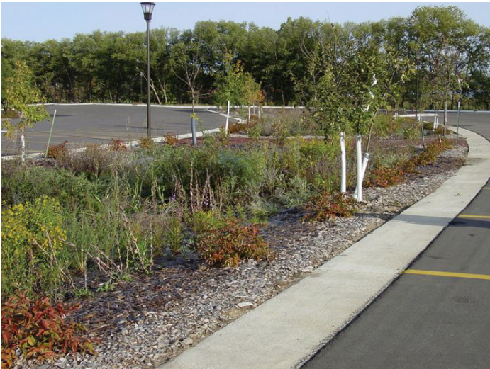
Photograph 4-9. Concrete edge acts as level spreader, distributing flow from parking lot as sheet flow to SCM.
