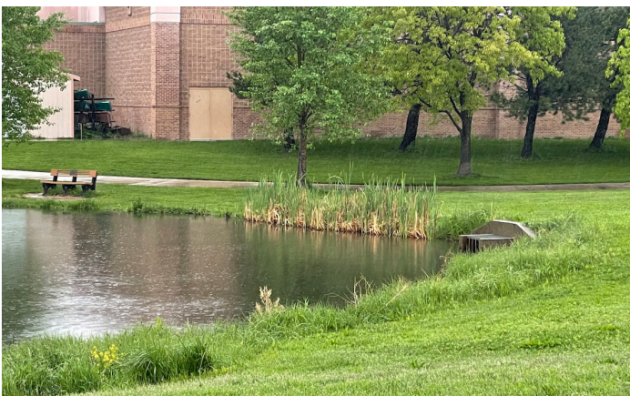
Photograph RP/CWP-7. This pond outlet structure is accessible and functional while not interfering with the overall pond aesthetic.
