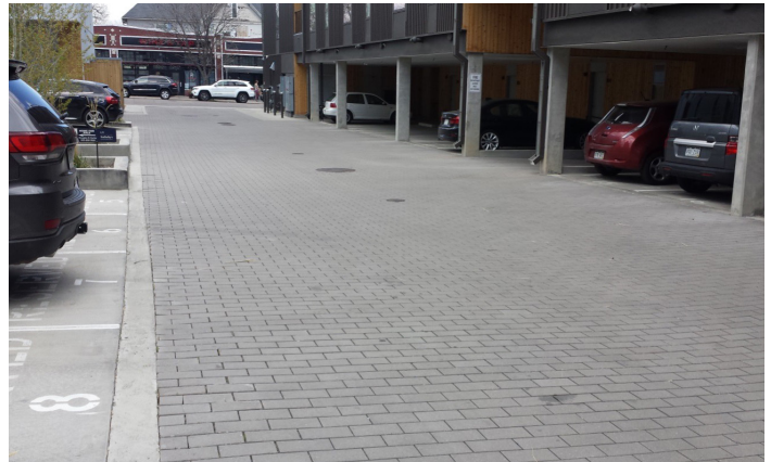
Photograph PPS-2. PICP in alley treats runoff from roof drains and adjacent parking spaces. A surface overflow path to the street provides drainage if the system is clogged or overwhelmed by runoff.
