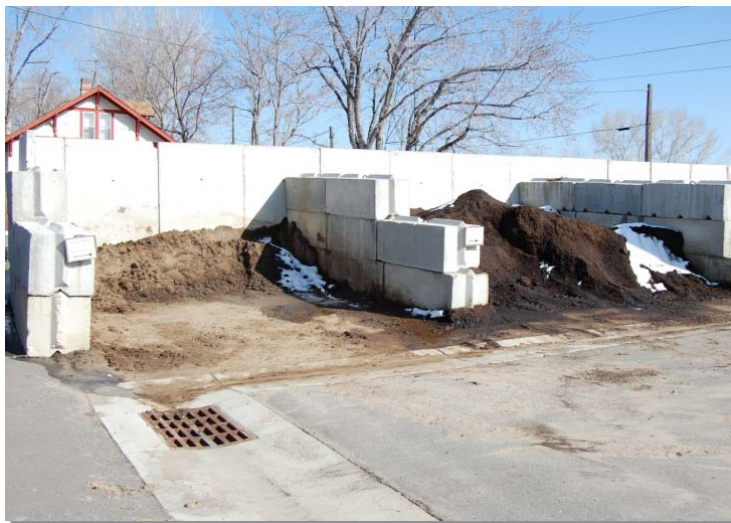
Photograph 5-1. This commercial materials storage area drains directly to a storm drain. Effective site design would have located this storage area away from a storm drain and directed runoff to a landscape bed or provided additional covering and containment that would both protect the material and reduce pollutant loading to the storm sewer.
