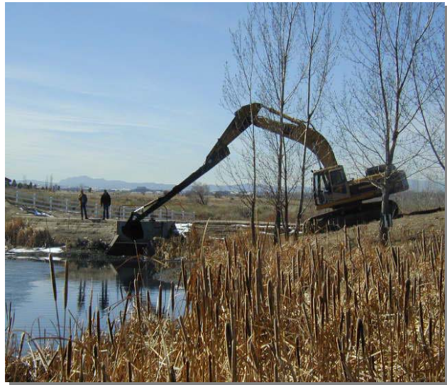
Photograph 6-1. Sediment removal from a forebay at the regional Shop Creek BMP System.
