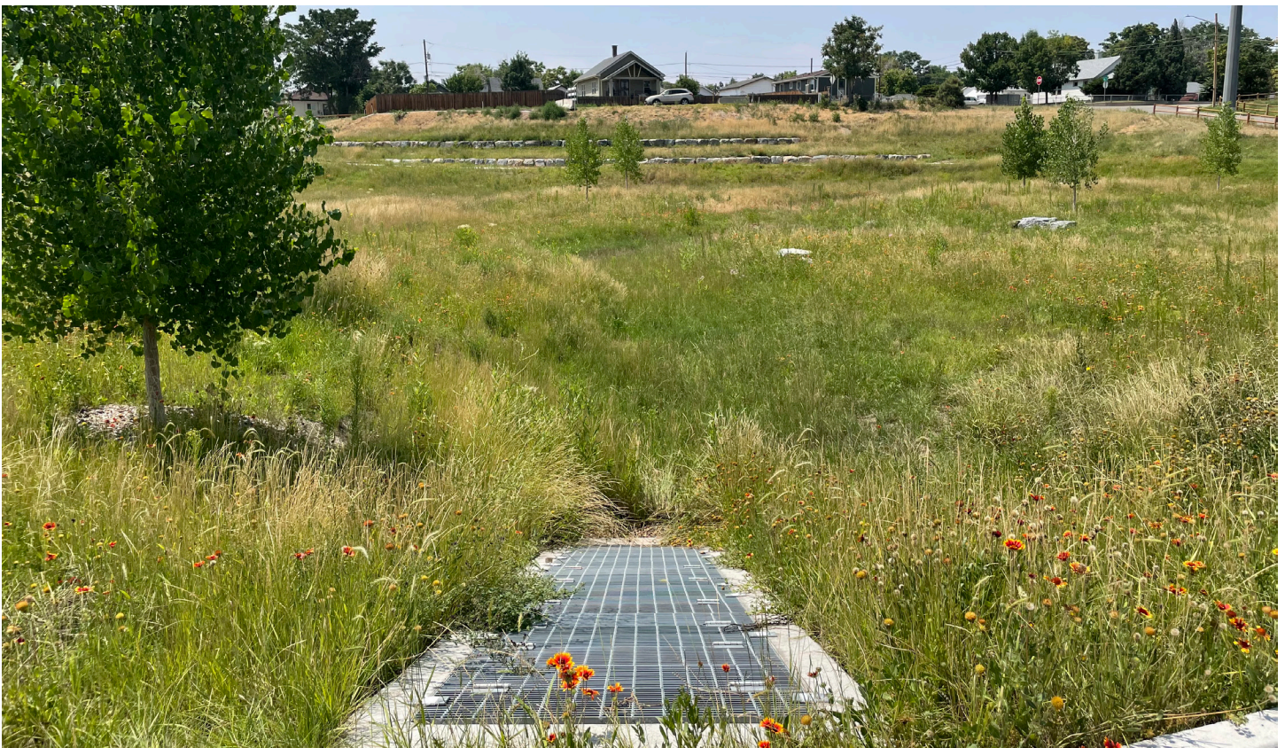
Photograph EDB-1. This EDB illustrates the use of a soft, meandering low flow channel and varied bottom grading with vegetation selected for the associated hydrologic conditions.
