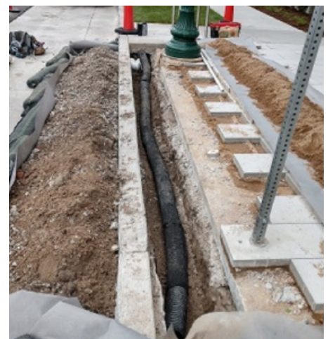
Photograph PPS-7. Perimeter barrier and trench with underdrain to protect street subgrade with adjacent PPS installation. Photo: Beck Group.
