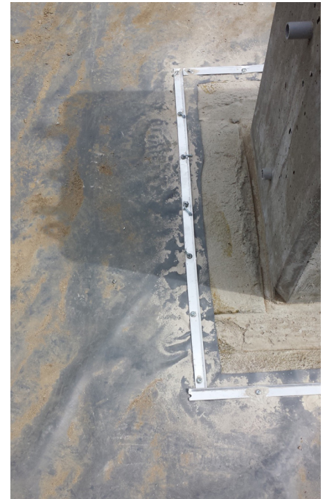
Photograph PPS-11. Geomembrane attachment to horizontal footing for light pole. Photo: Creative Civil.
