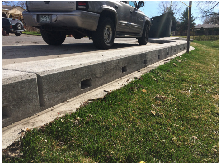
Photograph 4-7. Slotted or perforated curbs distribute pavement runoff and can function as a sediment forebay able to be maintained with a street sweeper.
