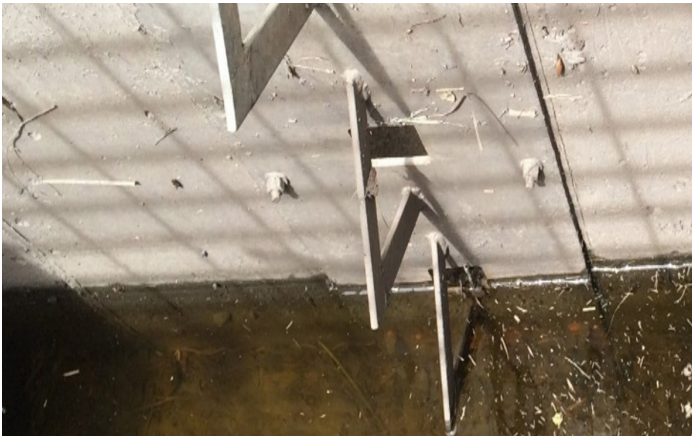
Photograph EDB-4. Where orifices are large enough to omit well screen, trash deflectors can be used in combination with standard bar grating to reduce the likelihood that debris will plug one or more orifice.
