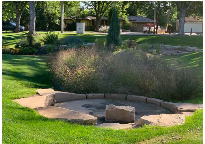
Photograph 4-15. Morse Park forebay provides energy dissipation with placement of a boulder, and the dense vegetation helps encourage sediment to stay in the forebay. This is an easily accessible area to remove sediment and trash, and it provides even distribution of flow to the SCM.
