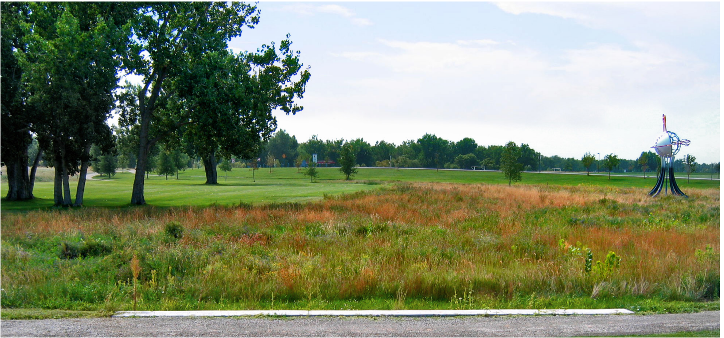
Photograph 4-13. Level spreader at Aurora Sports Park evenly spreads flow to the wetland area downstream.
