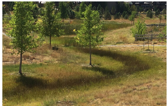
Photograph RPA-6. Dense vegetation in this 5% sloping swale provides the roughness to resist erosion and slow, filter, and infiltrate runoff. Photo: Muller Engineering.
