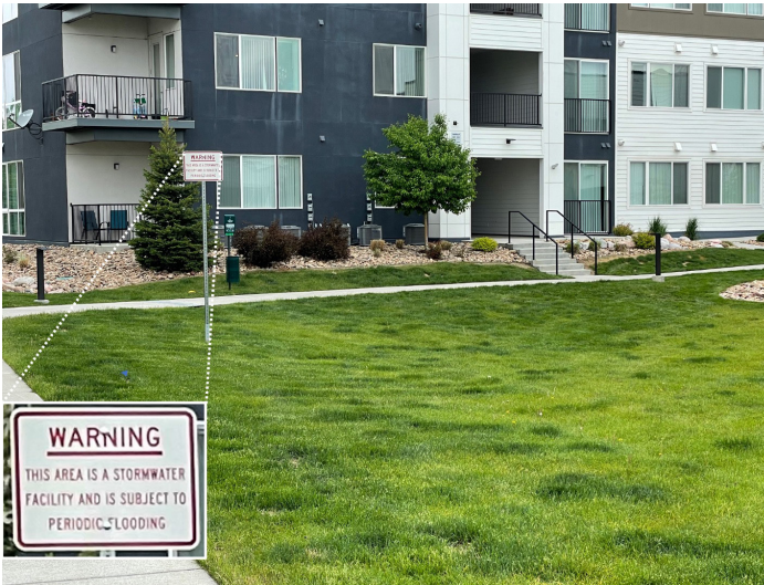
Photograph RPA-7. RPA in multi-family residential neighborhood. Sign warns of periodic flooding which helps establish expectations for periodic temporary ponding, while providing a safety warning. Photo: WWE.
