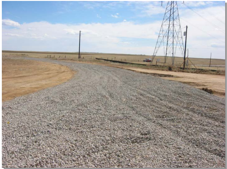
Photograph SCR-1. Stabilized construction roadway.
