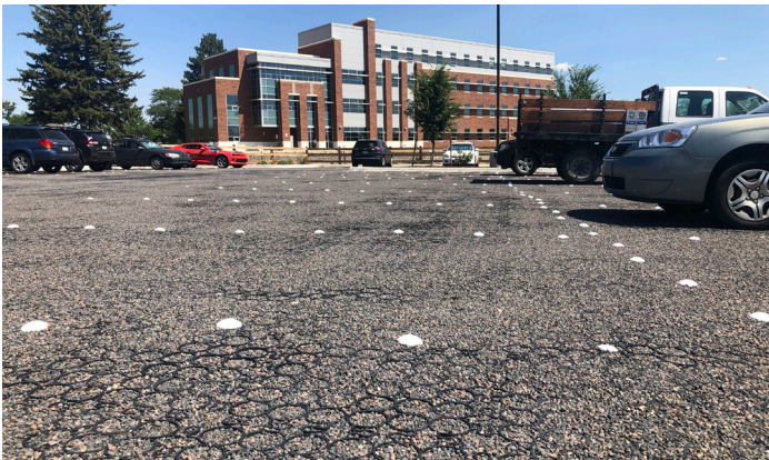
Photograph PPS-5. PGP with grid for containment of surface materials to minimize potential for rutting. Photo: True Grid.
