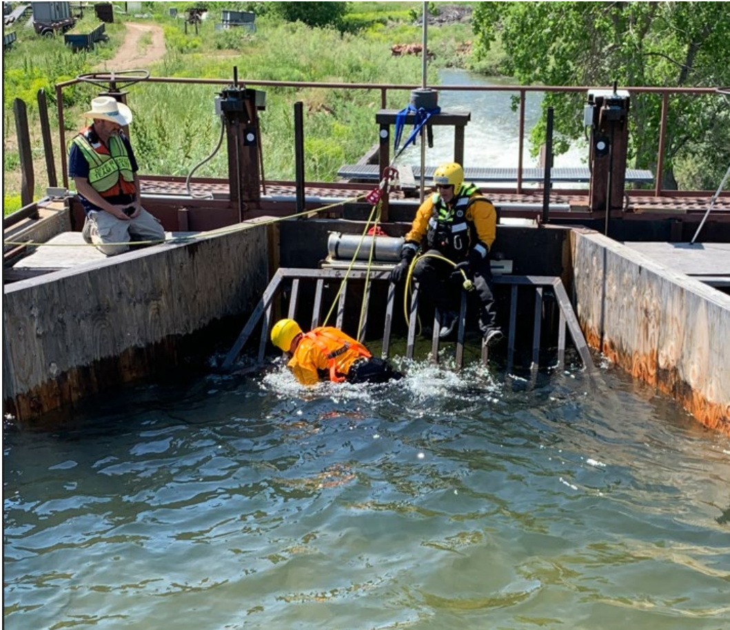
Figure 8. Test 2 (MHFD 1:1 (H:V) Grate, 48-inch Diameter)
