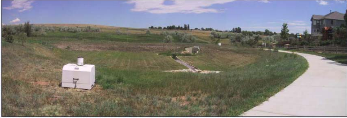
Photograph 1. Grant Ranch EDB with inflow sampler box shown in the foreground.
