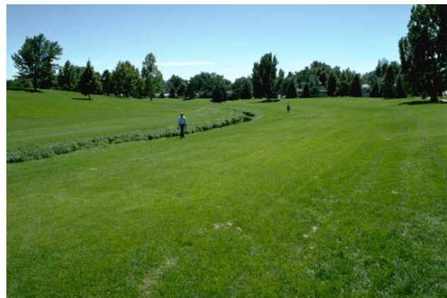
Photograph 3-6. A wide, open waterway carries floodwater at modest depths while maintaining low velocities to inhibit erosion.
