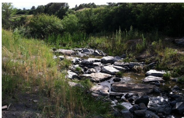
Photograph 8-8. Proactive stabilization at McMurdo Gulch, constructed with little disturbance to the existing channel.
