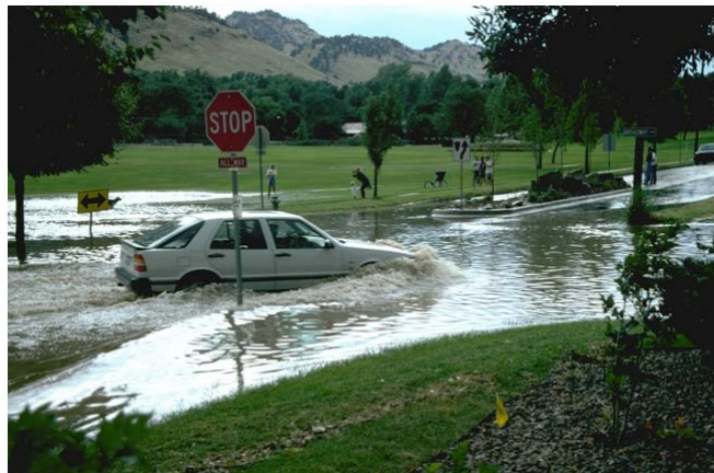
Photograph 3-2. UDFCD drainage criteria are aimed at respecting the needs of safe, unimpeded traffic movement. This intersection represents a long-standing drainage problem needing a solution.
