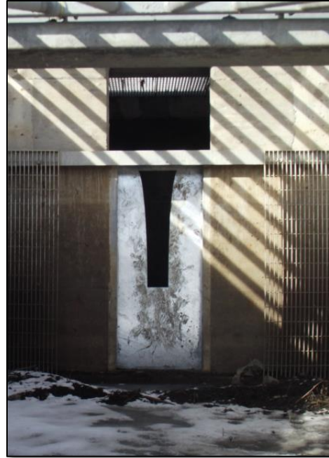
Figure 16. Actual installation of (left) water quality orifice plate, and (right) elliptical slot weir for the Northfield Detention Basin.
