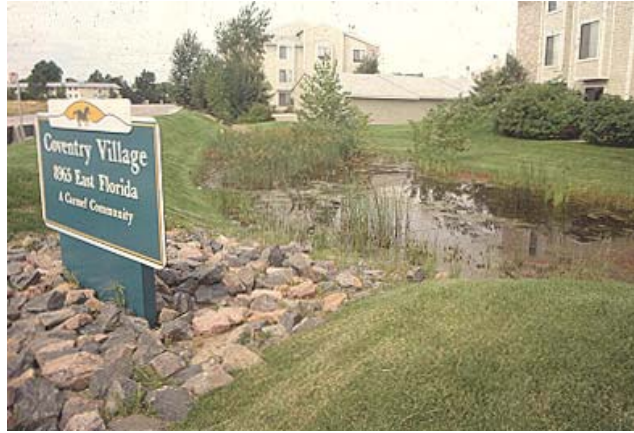
Figure 13. A detention basin with a pond at an apartment complex in Aurora, Colorado.
