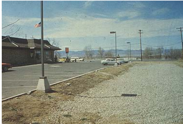
Figure 14. A dry detention basin next to a MacDonalDs Hamburger facility in Littleton, Colorado
