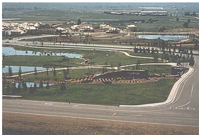
Figure 12. Photograph of a portion the Rock Creek development in 1996 in Superior, Colorado.
