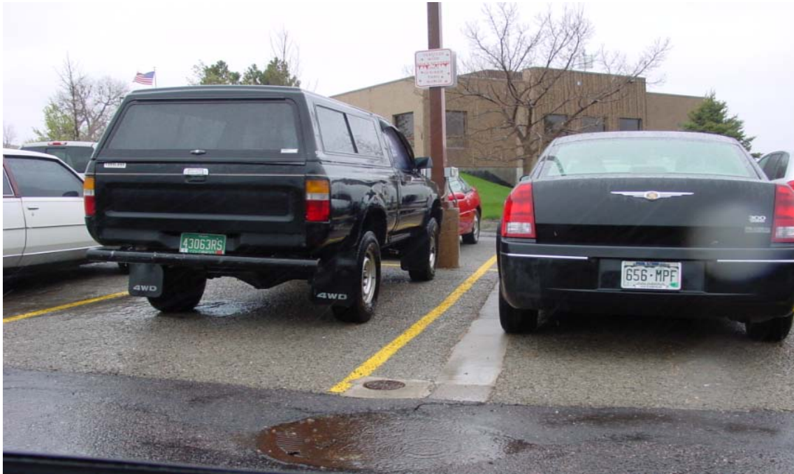
Photograph 1. Pervious concrete at Lakewood Maintenance Facility
