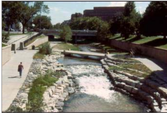
Figure 4. A grouted boulder grade control structure in combination with a trail crossing along Cherry Creek at a highly developed central city site.
